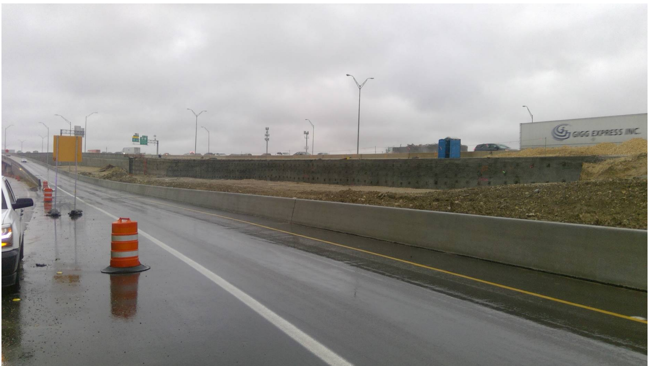
Soil nail wall 2100
