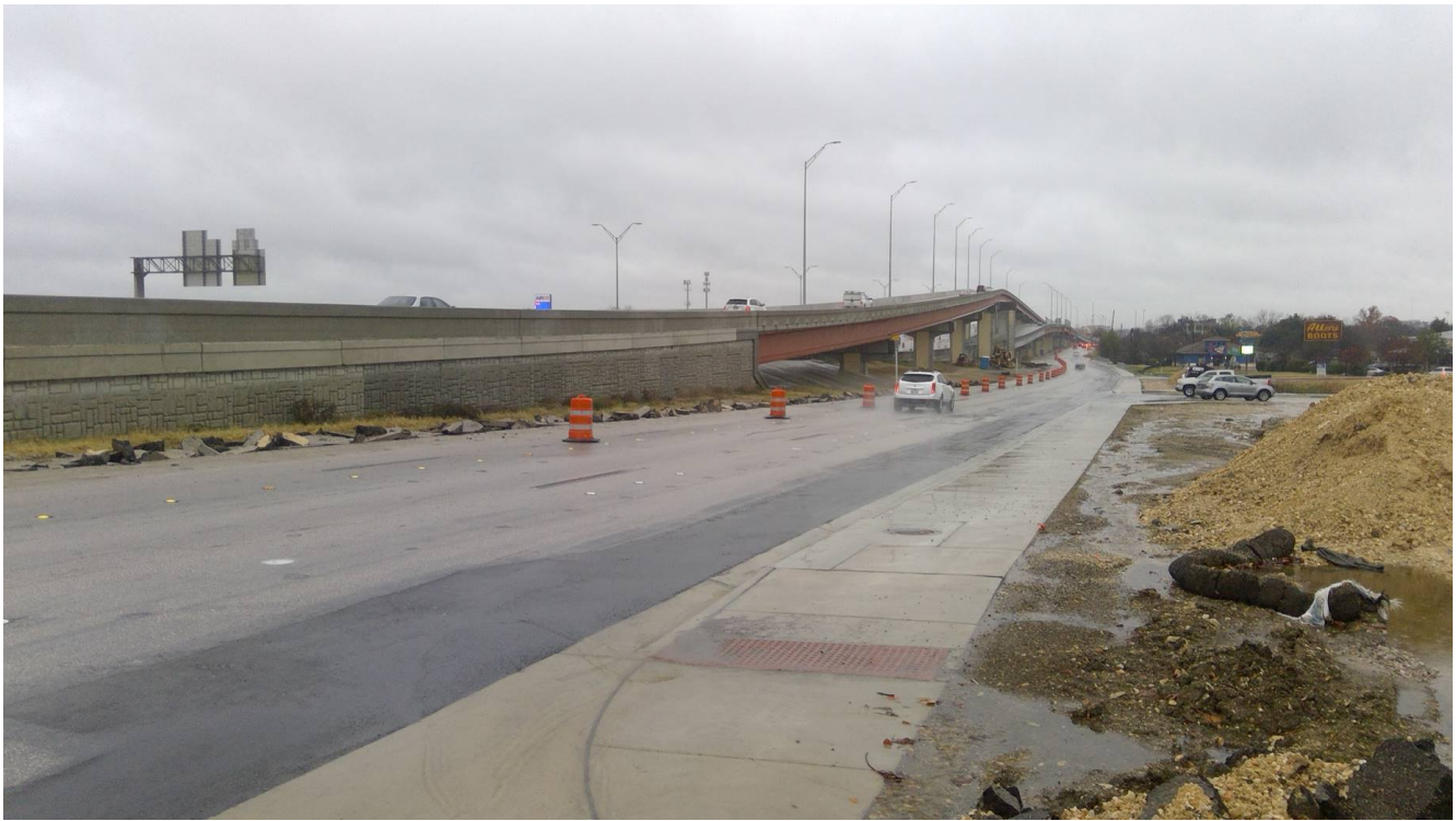
Northbound frontage road curb
