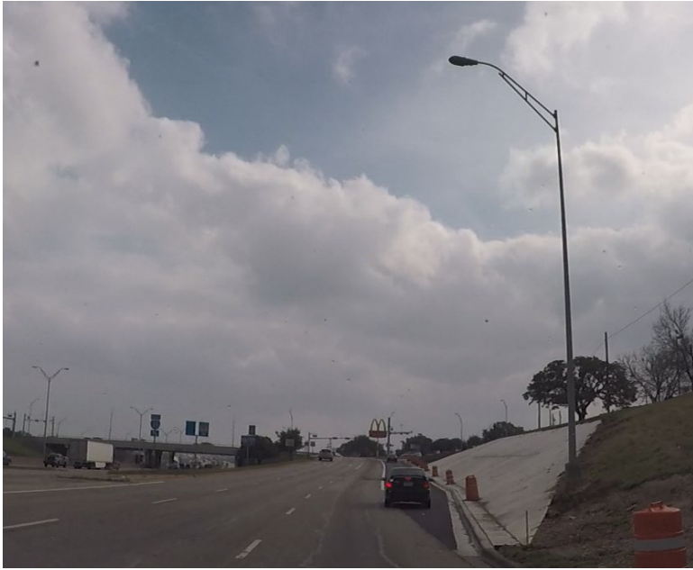
Southbound frontage right turn lane at RM 620
