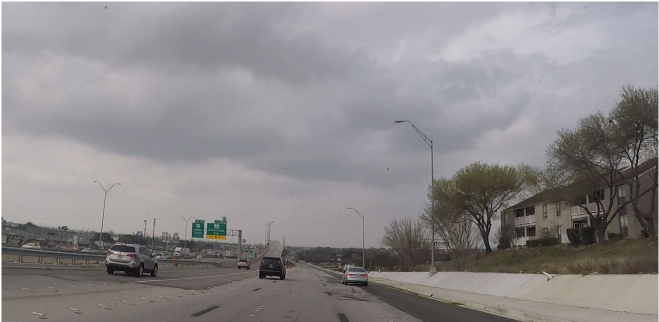
Northbound frontage road final configuration
