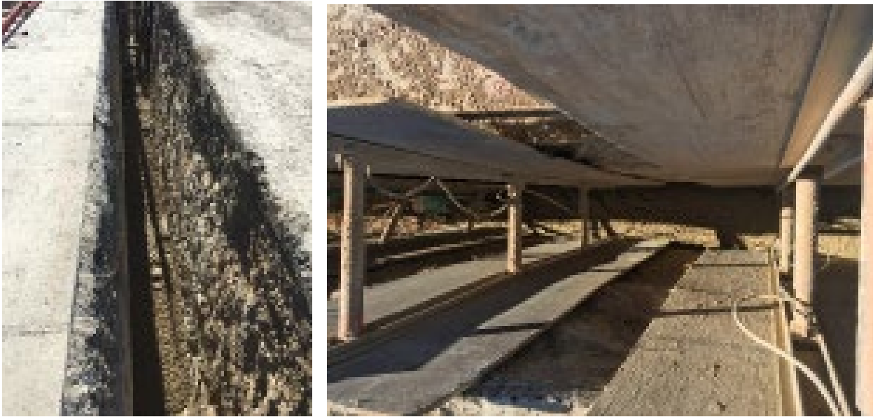
Backfilling City of Austin sanitary sewer trench with flowable fill line
