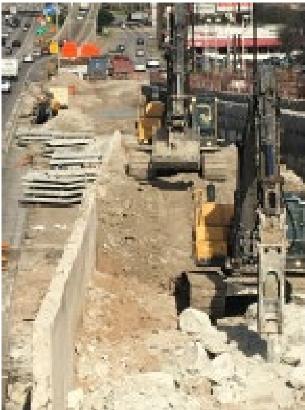
Excavation for northbound collector distributor at rock wall nail wall
