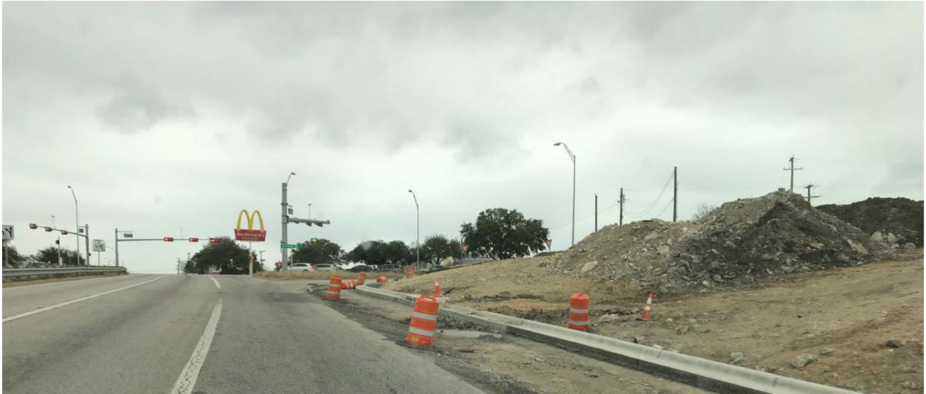
Southbound frontage right turn lane at RM 620
