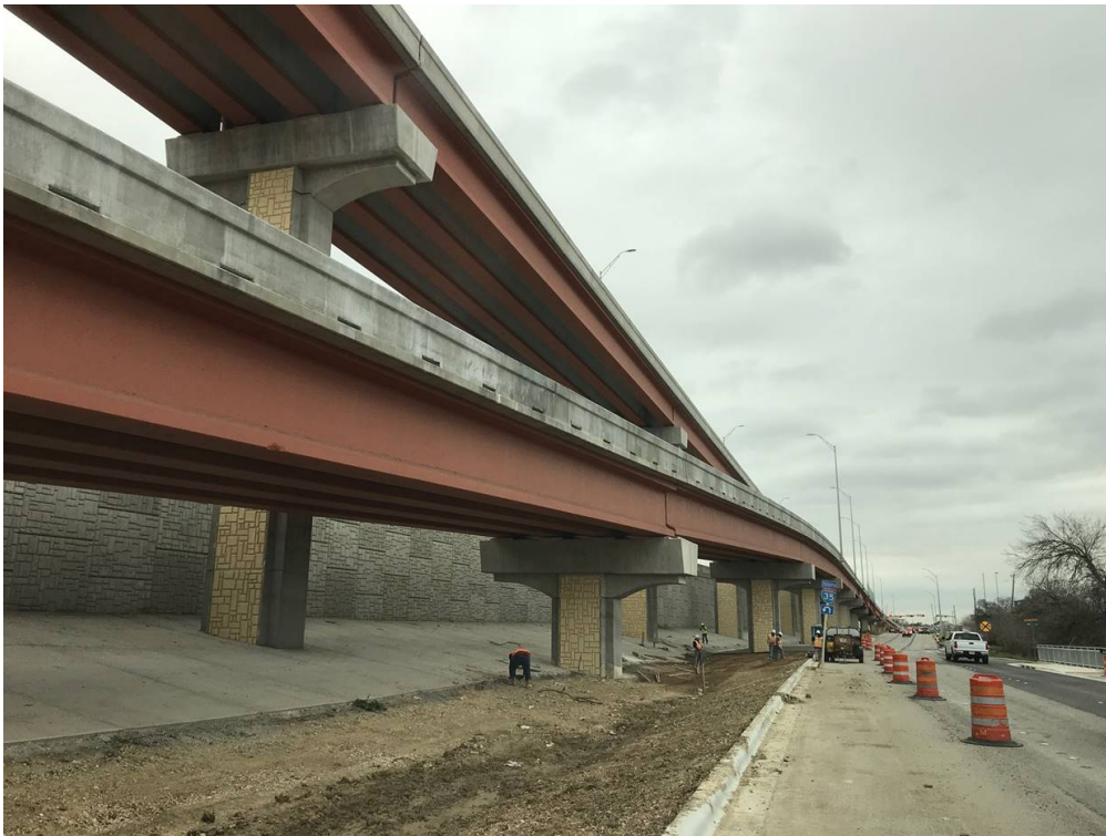
Soil nail wall 2100
