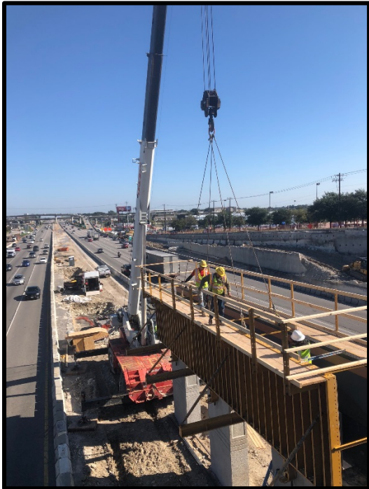
Setting cap forms in the center of I-35 for the St. Johns south to north U-turn bridge
